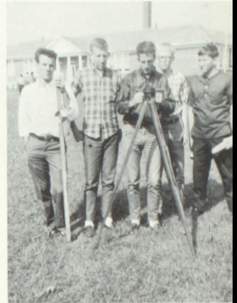
Terracing and drainage is of major importance in our Vocational agricultural program.
