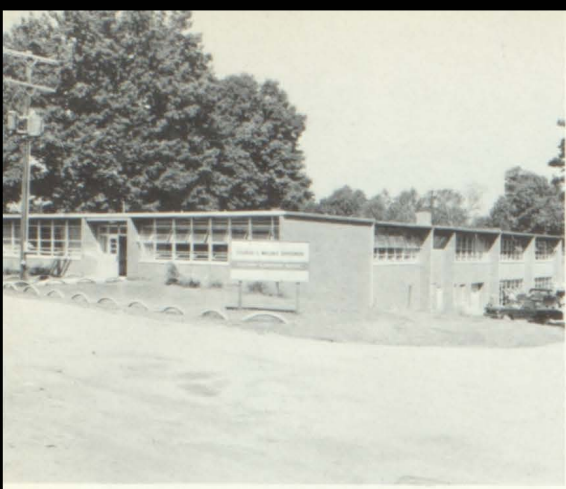
New Elementary Building
