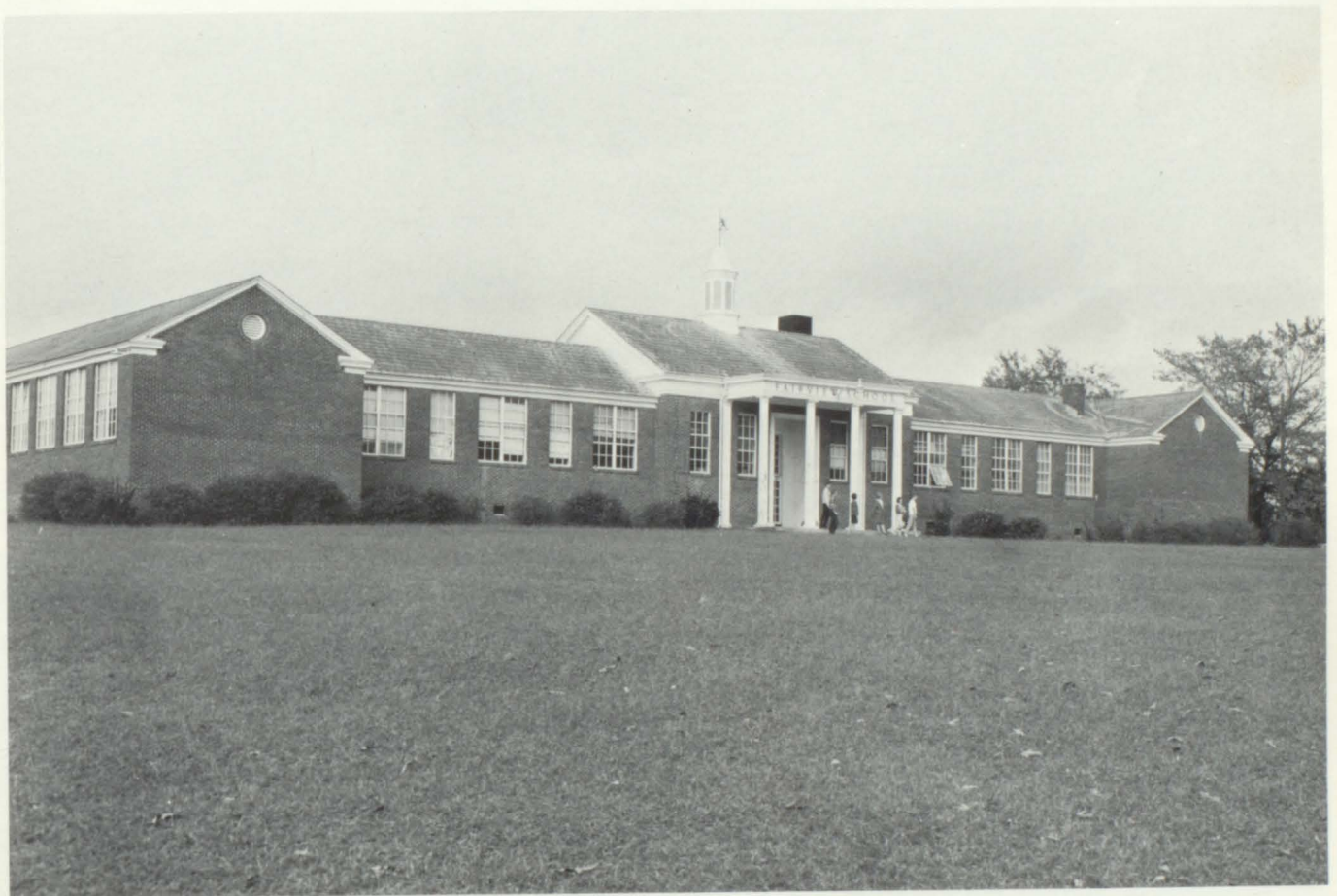
High School Building
